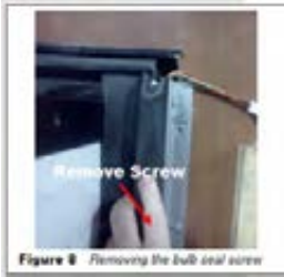
Figure 8 Removing the bulb seal screw
